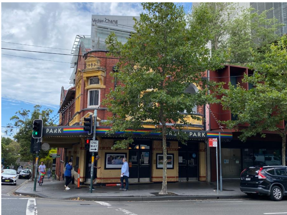
Figure 2: Site viewed from Victoria Street facing east
