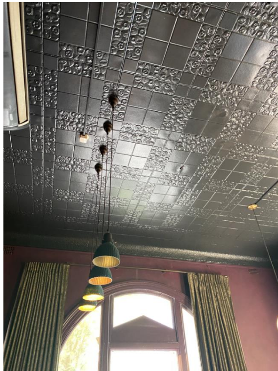
Figure 8: View of ground floor level ceiling
